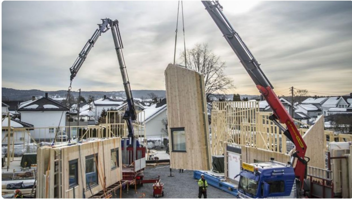
Figure 11. MMC assembly stage by Norwegian company Optimera (SAINT-GOBAIN, 2022)
