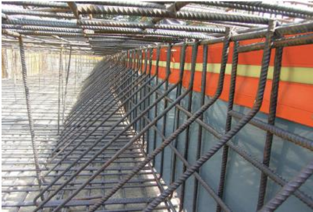
Figure 7. DRYset crack inducing unit
