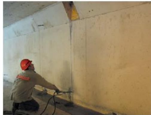
2. Injection of crack-inducing unit
