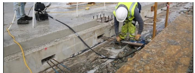
Figure 2. Post tensioning of the GeoStruct Reactive Slab System
