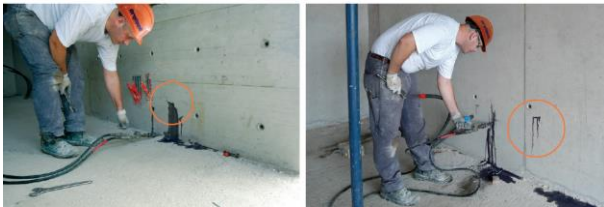
Figure 3. Filling and pressure sealing the joint with DRYflex resin
