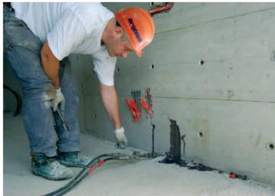
1. Injection of cold joints and movement joints
