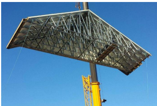
Figure 1: Prefabricated Modular LGS Roof Truss Element Being Lifted into place
