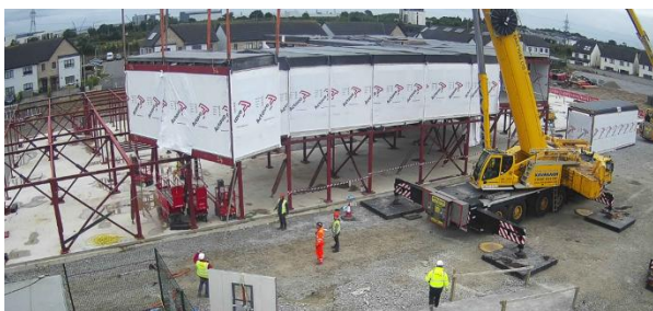
Figure 2: Module installation in progress on site.
