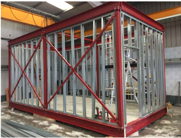
Figure 1: Modular unit without finishes
