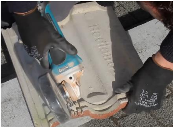
Figure 6: Tile Notching
