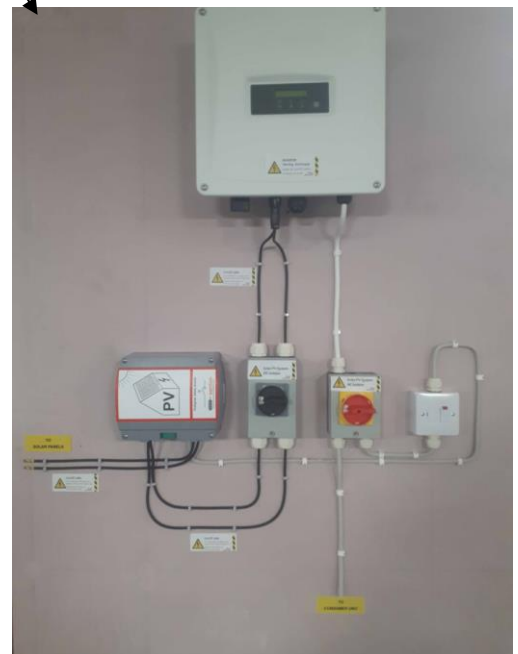
Figure 2: Roof fixing and inverter/electrical isolators layout
