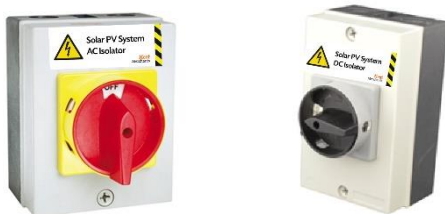
Figure 10: DC and AC Isolators
