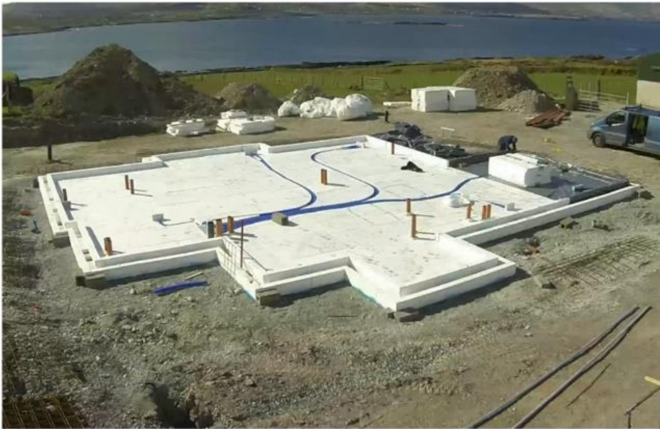
Figure 1 - KORE Insulated Foundation System before DPM and Concrete
