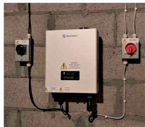
Figure 15: Installed inverter with electrical isolators
