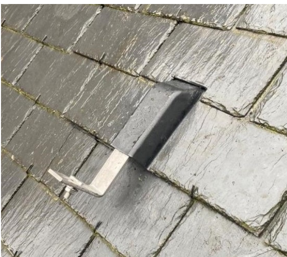
Figure 8: Solarflash on slate roof
