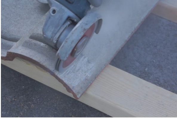
Figure 6: Tile Notching
