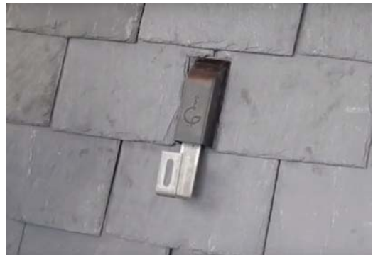
Figure 8: Finished Slate Flashing Example
