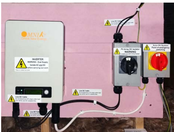
Figure 13: Installed Inverter with Electrical Isolators
