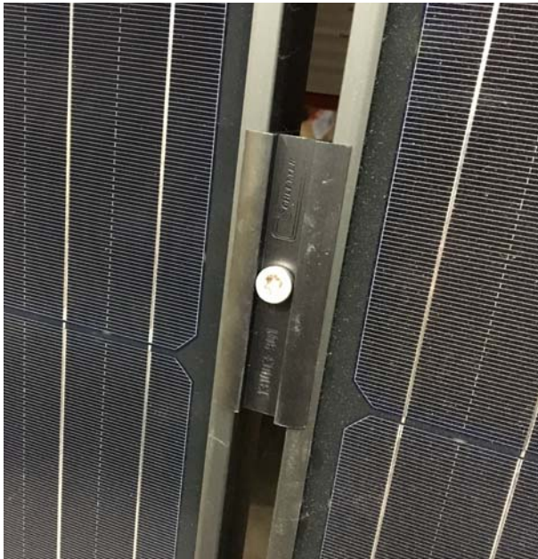
Figure 4: Module Clamp
