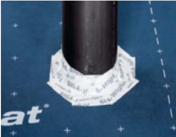
Figure 9: Siga Cable Sealing Example
