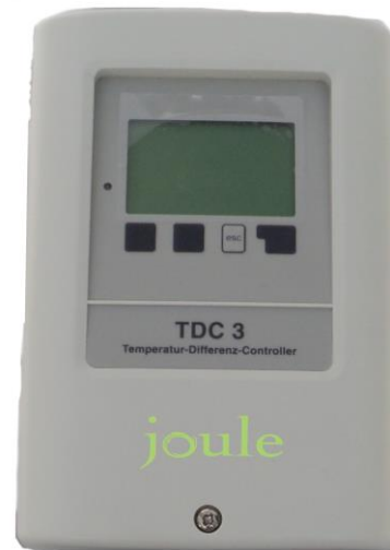
Figure 15: Joule Control Panel
