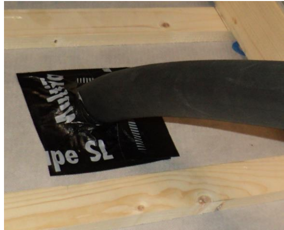
Figure 10: Sealing of Roof Underlay
