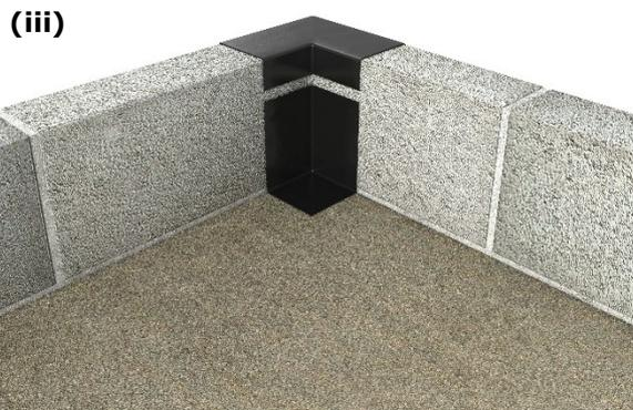
Place the internal corner section neatly into the inside corner.
