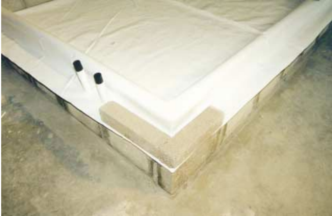
Fig 4: Dura Skrim 15 WW Radon Resisting Membrane with Top Hat seals on service ducts
