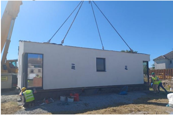
Figure 1: Positioning a module on substructure
