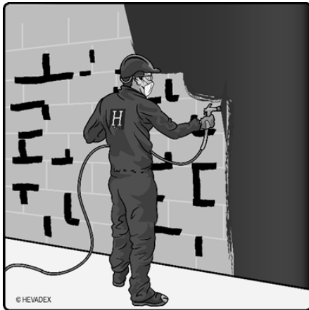
Figure 3: Application of BLOWERPROOF® onto walls.
