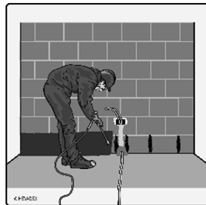
Figure 7: Application of BLOWERPROOF® at floor to wall junctions.
