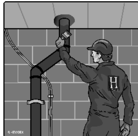
Figure 5: Application of BLOWERPROOF® at pipe penetration.
