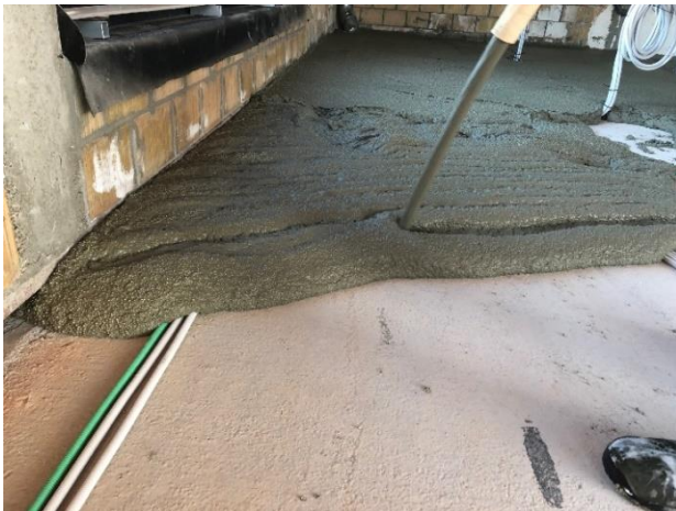
Figure 3: baseTherm® pumping and levelling
