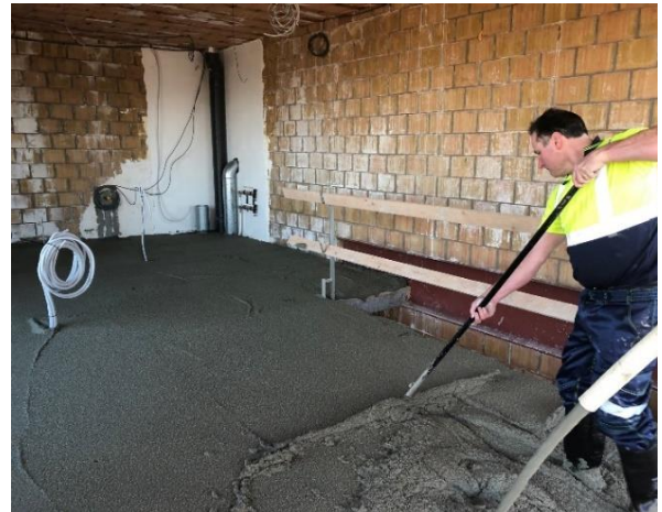
Figure 3: baseTherm® pumping and levelling
