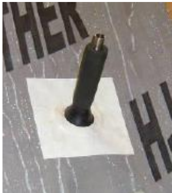
Figure 7: Sealing of the Roof Underlay using the Glidevale self adhesive sealing collar
