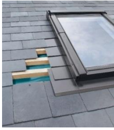
Figure 14: ELV Roof Flashing
